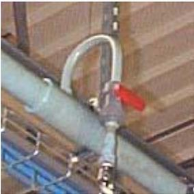
The traditional method is to install an upward loop.
